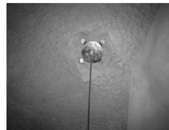
(c) Pressure cell installation
