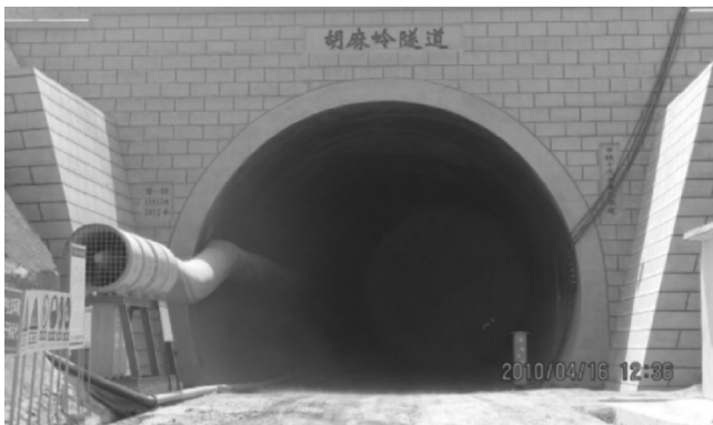
Figure 1. North portal of the Hu Maling tunnel
