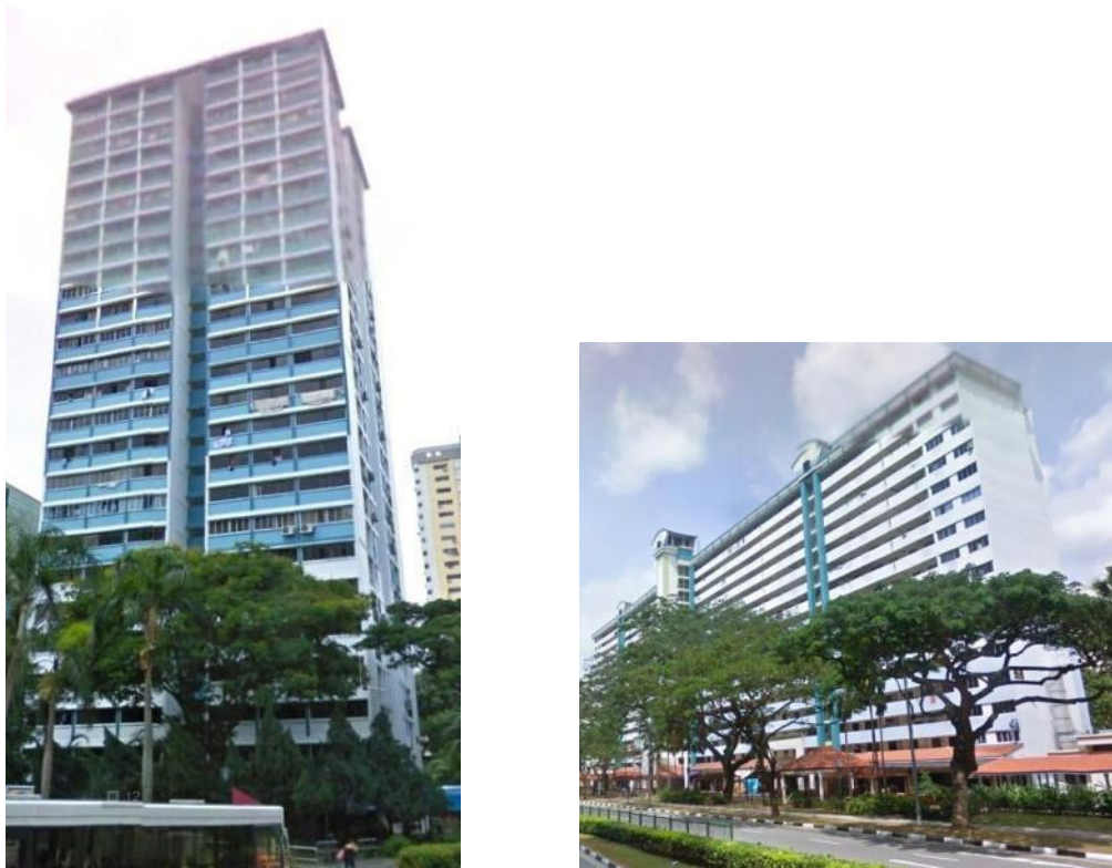
(a) (b) Figure 2-2 Photos of (a) 25-storey point block; (b) 16-storey slab block
