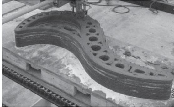
Figure 8. Concrete printing at Loughborough University (Le et al., 2012)
