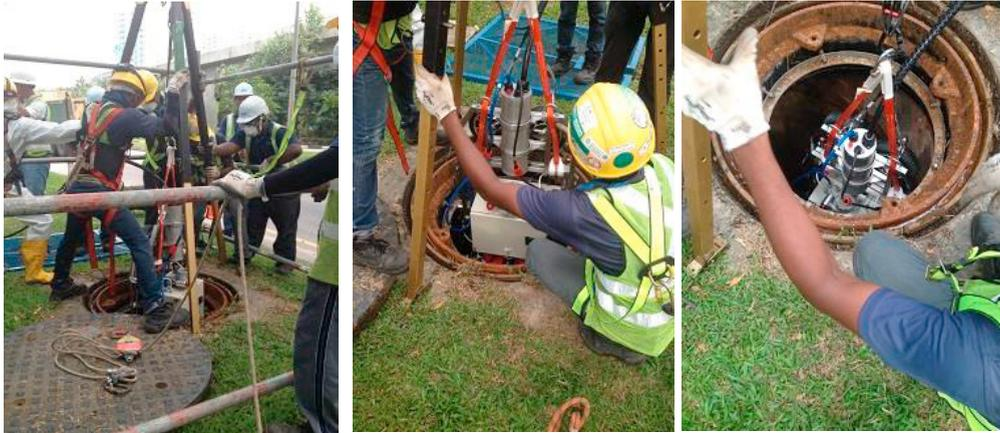
Fig. 3. Compact Mobile Robot for Sewer Inspection.
