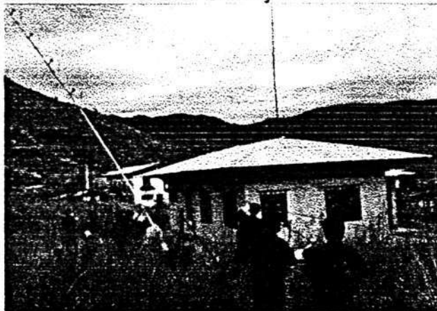
Radio NYAB Building
