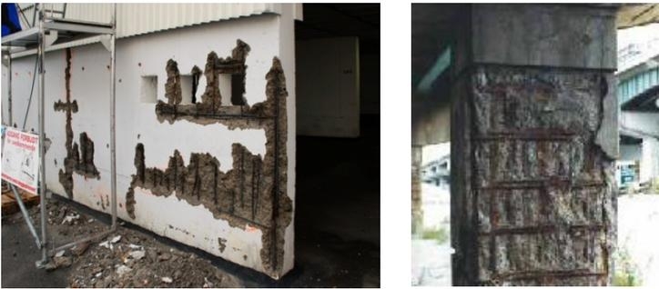
Figure 1: Corrosion of transverse rebars.
