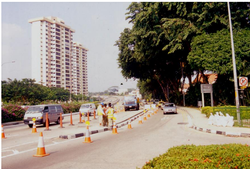
Figure 1.2 Temporary restriction on access to median due to ground surface settlement
