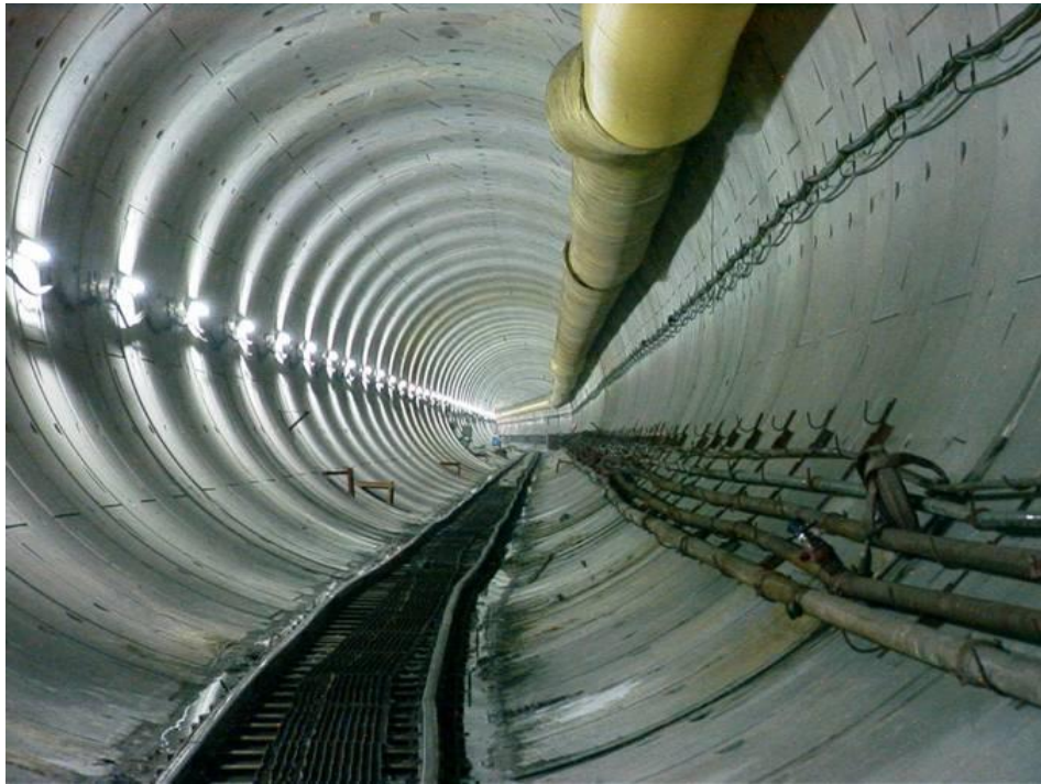
Figure 1.6 Jointed precast segmental linings
