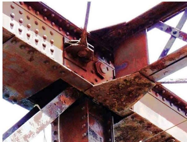
(b) Steel connections
