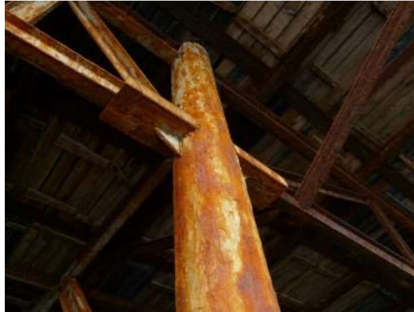
(a) Steel columns
