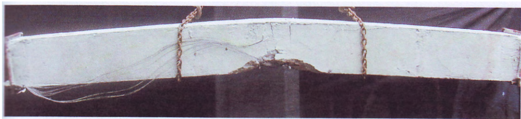
Figure 6.20 Failure mode of restrained composite column CC10
