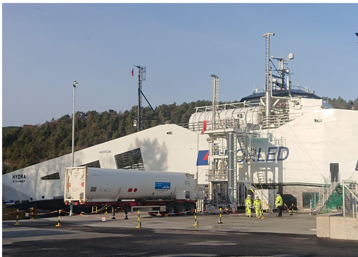
Figure 3-12: Mobile bunkering tower for LH2 transfer to MF Hydra ferry
