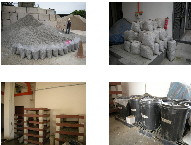
Figure 3.5 Material preparations for batching of concrete
