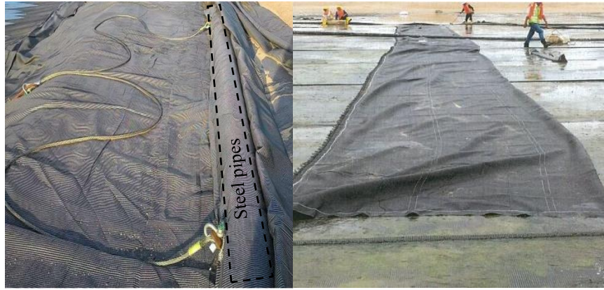
(a) Placement of geotextile and geotextile tube
