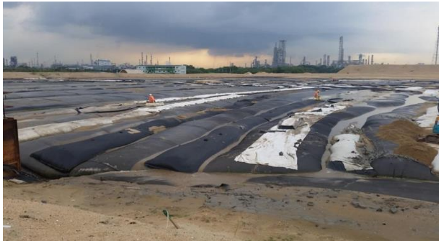
(b) Installation of sand berms using geotextile tubes
