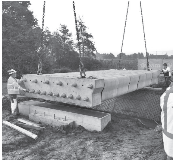
Fig. 7 Hoisting the bridge into position.
