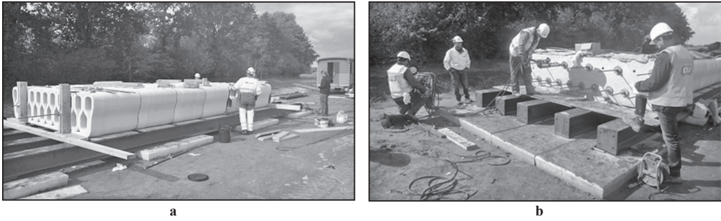
Fig. 6a, b On-site assembly and prestressing.
