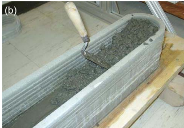
68 Fig. 1 Contour Crafting [13] : (a) schematic drawing of printing nozzle; (b) formation of composite 69 structure. Reproduced from Ref. [13] with permission from IAARC.
