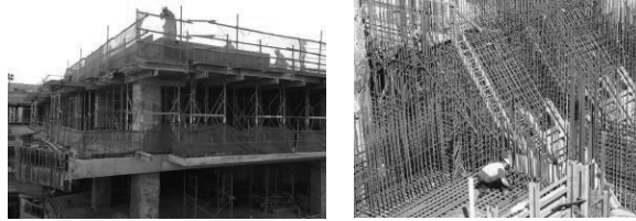
Figure 2. Example of formwork and the complex reinforcement in civil construction work.
