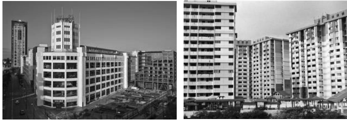
Figure 1. The first Philips building in Eindhoven, 1909 (left) and present concrete buildings like some colorful housing in Singapore 1977 (right).
