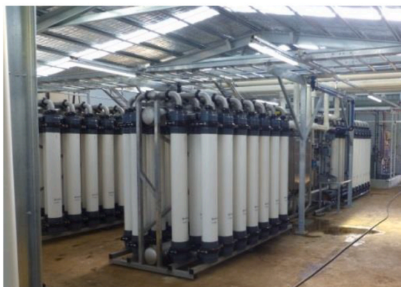
Fig. 7. Full-scale hollow fiber nanofiltration at Ringarooma Valley, Australia. A) Picture of the hollow fiber nanofiltration skids, reproduced from [144] B) Schematic overview of the treatment scheme, image based on information in [144].
