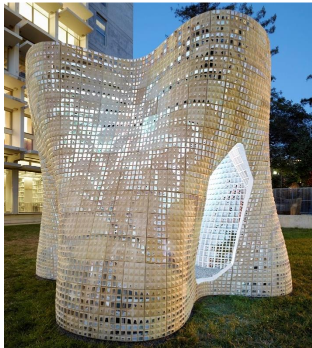
Figure 2.12. Structure printed in modular that has different light permeability [40].
