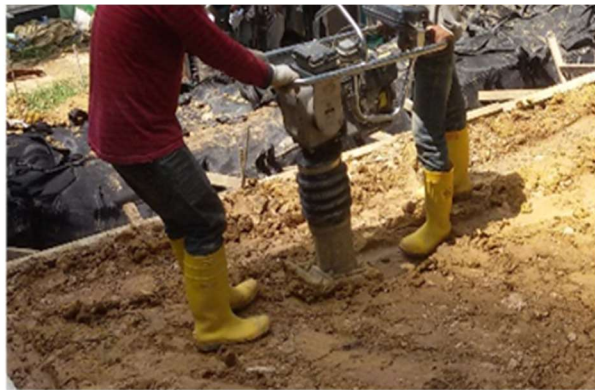
(b) Compaction of residual soil behind Capillary barrier
