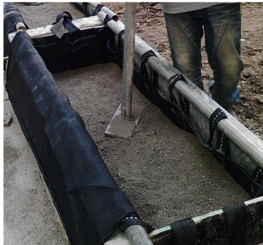
Figure 23: Filling and compaction of fine RCA/fine RAP inside geobag
