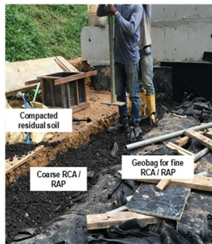
(c) Placement of coarse RCA/coarse RAP
