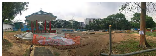
Figure 7. Yunnan Garden during refurbishment. © Seide, Reinhuber, Williams. 2018
