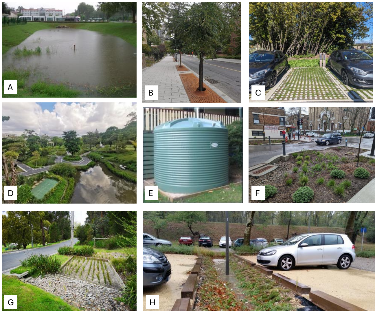
487 Figure 5. Examples of stormwater control measures. Stormwater infiltration pond, Villeurbanne, France 488 (A), stormwater runoff-irrigated street trees, Montreal, Canada (B), Porous pavement, Valence, 489 France (C), Wetland and rain-garden, Singapore (D), Rainwater tank, Melbourne, Australia (E), 490 Streetscape rain-gardens (F & G), Montreal, Canada and Melbourne, Australia, Carpark 491 infiltration swale, Villeurbanne, France (H). Photo credits: Frédéric Cherqui. These examples
