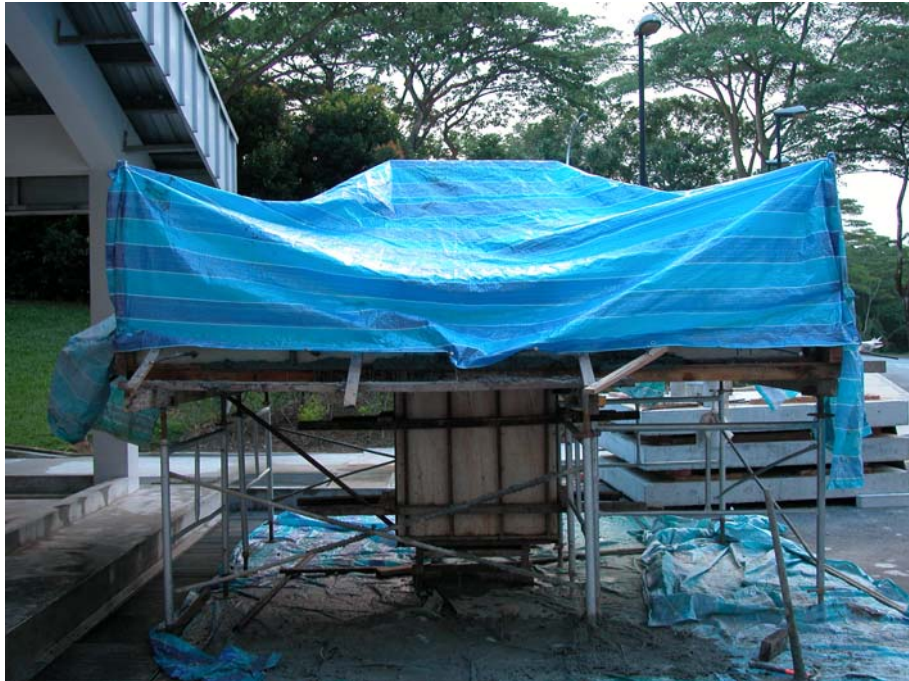
Fig. B.3 Curing of concrete
