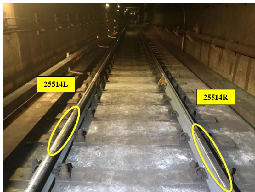
Figure 7-11: 2-clad rail specimens installed at Redhill-Tiong Bahru [CH 25514L & CH 25514R]
