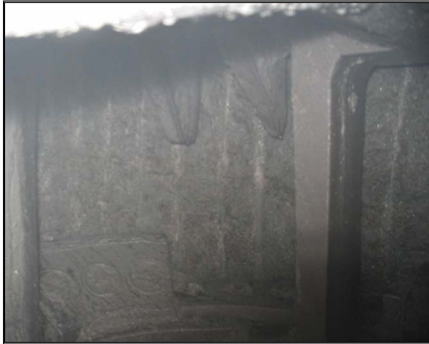
Figure 6.22 Tunnel face in N1877, T06
