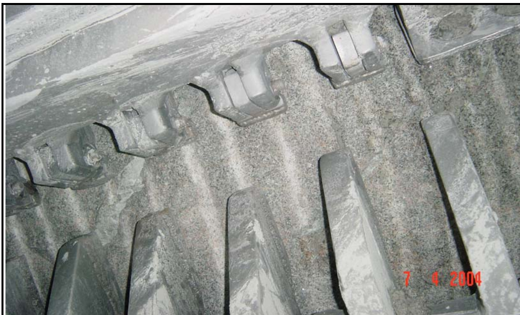
Figure 6.12 Tunnel face at upper right opening (North Ring 2734 in T05)
