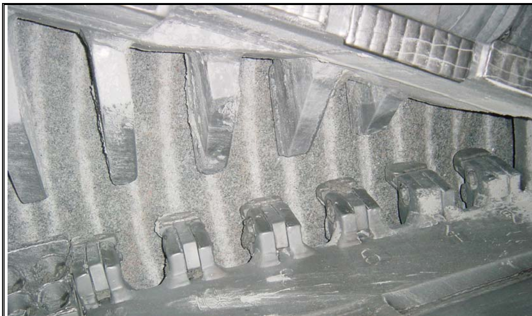
Figure 6.13 Tunnel face at upper left opening (North Ring 2734 in T05)
