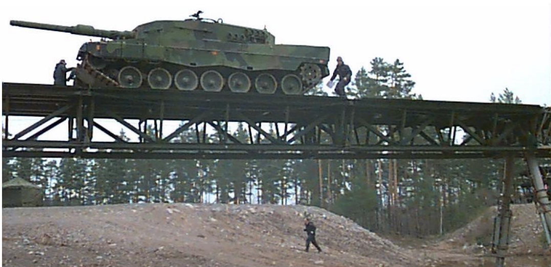
Figure 1.2: Fast Bridge 48 Military Bridge, Sweden (Collin and Johansson, 2006)
