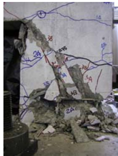
(d) Buckling of reinforcing bars at right bottom column at DF = \pm 4
