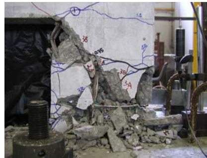
(e) Damage of bottom right column at DF = \pm 5
