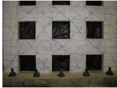
(b) Diagonal cracks at DF = \pm 3
