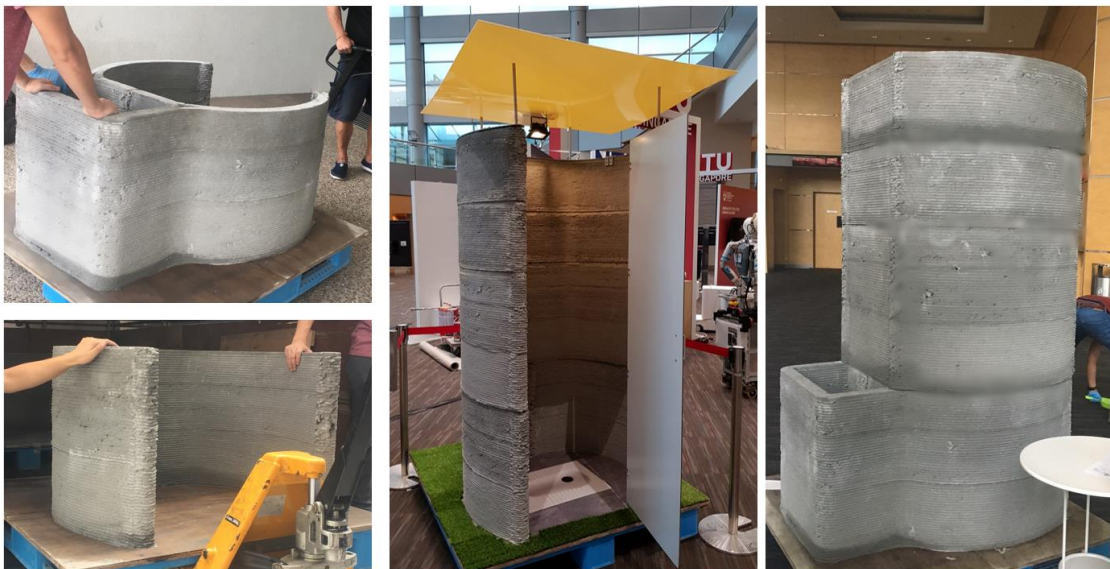
Figure 6.32 Snapshots of 3D concrete printed modular toilet unit
