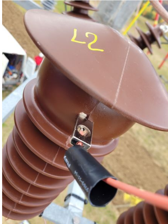
Figure 2.3: A high voltage CD shot on location.
