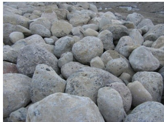
Figure 2-12: Close-up of Riprap
