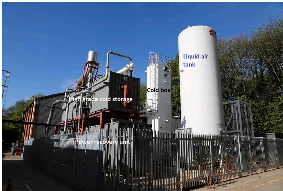
Fig. 16. High grade cold storage used in a 350 kW/2.5 MW h LAES pilot plant at the University of Birmingham, UK [19].
