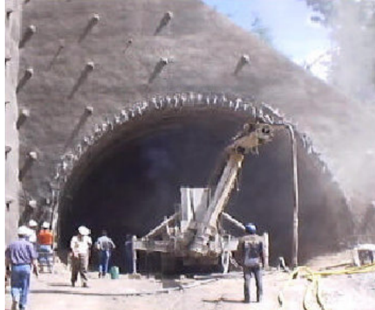
Figure 3-7. Grouting and excavation.
