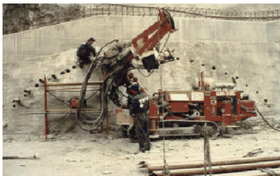
Figure 3-5. Drilling of holes.
