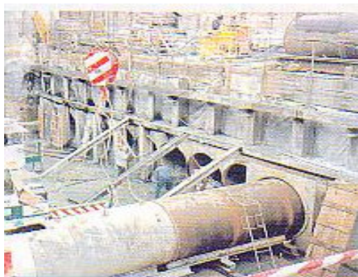
Figure 2-15. Pipe roof project.
