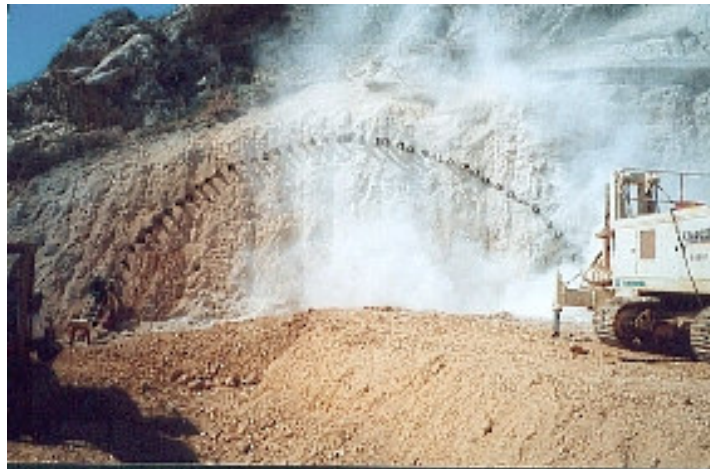
Figure 2-5. Forepoling method used for tunnel excavation in Greece. (Zeccos, 2002)
