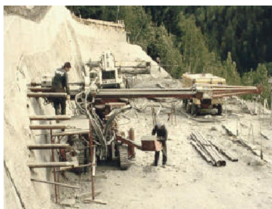
Figure 3-6. Insertion of steel pipes.
