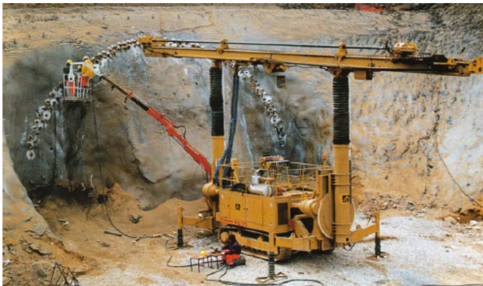
Figure 2-6. Forepoling rig (Rotex OY)
