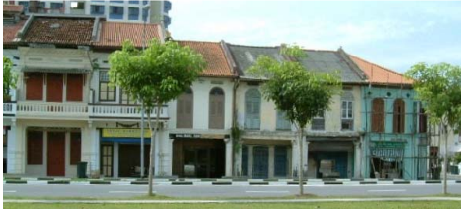
Figure 5.9 Typical Shop Houses C706A
