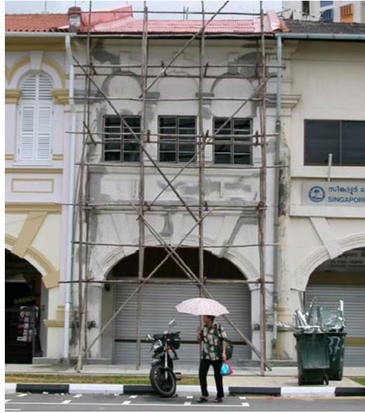
Figure 5.12 Repairing on the Infill Frame Structures at C706 e-n Shop Houses
