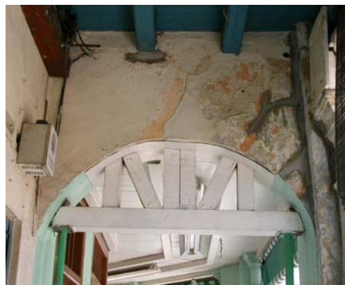
Figure 5.11 Protection of Arch
