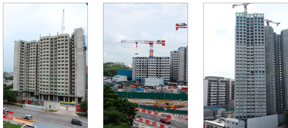
Figure 1. Images that depict PPVC buildings under construction.
