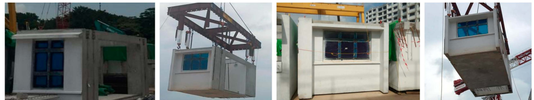
Figure 2. Images of PPVC modules taken from different angles.
