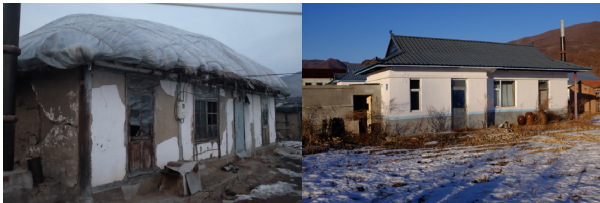
Figure 1: House in the old settlements and new house rebuilt by the government
