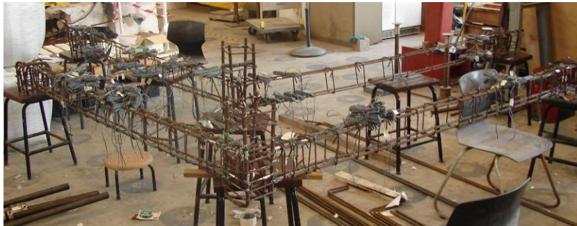
Fig. 3.17: Typical reinforcing cages
