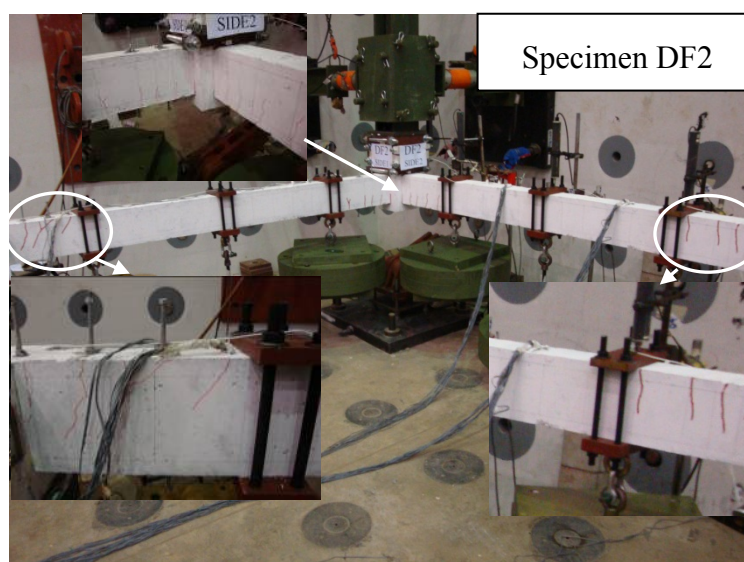
Fig. 6.12: Observed crack pattern of DF2 after test
