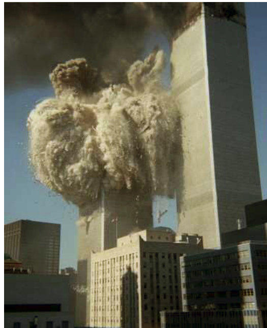
Fig. 2.3: World Trade Center under progression collapse ( http://www.solcomhouse.com/Worldtradecenter.htm )
