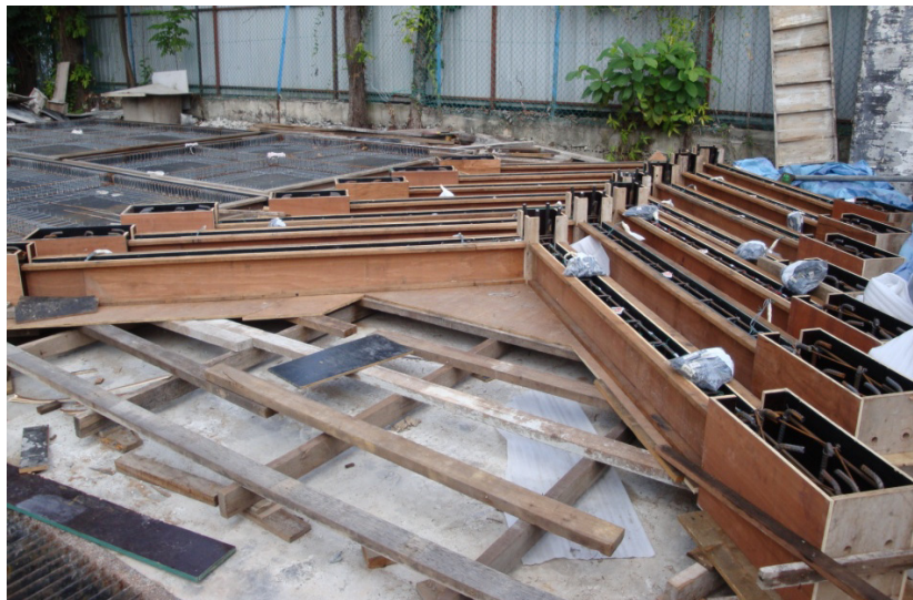
Fig. 3.18: Formwork with reinforcing cages
