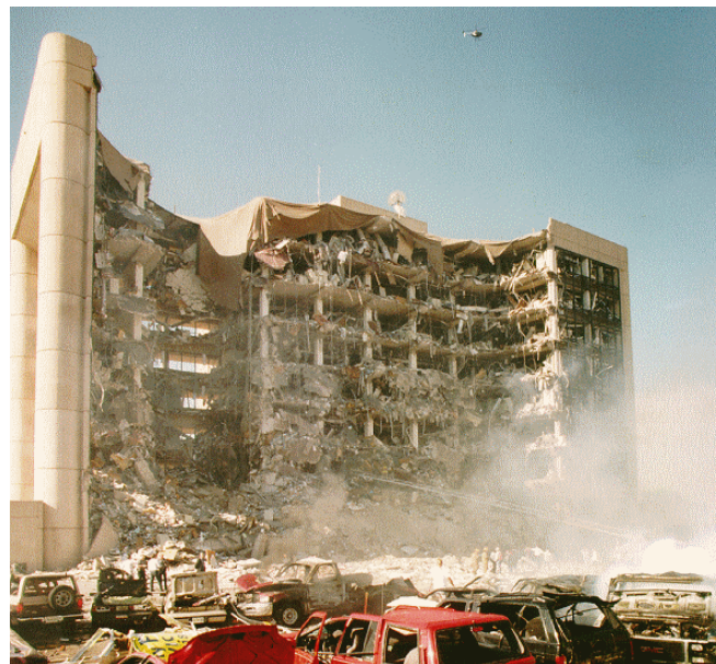
Fig. 2.2: Murrah Federal Building after collapse ( http://en.wikipedia.org/wiki/Oklahoma_City_bombing )
