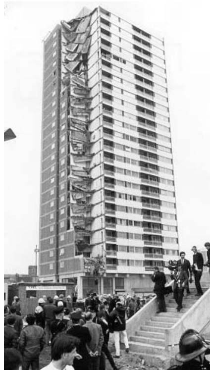
Fig. 2.1: Ronan Point Apartment after collapse
