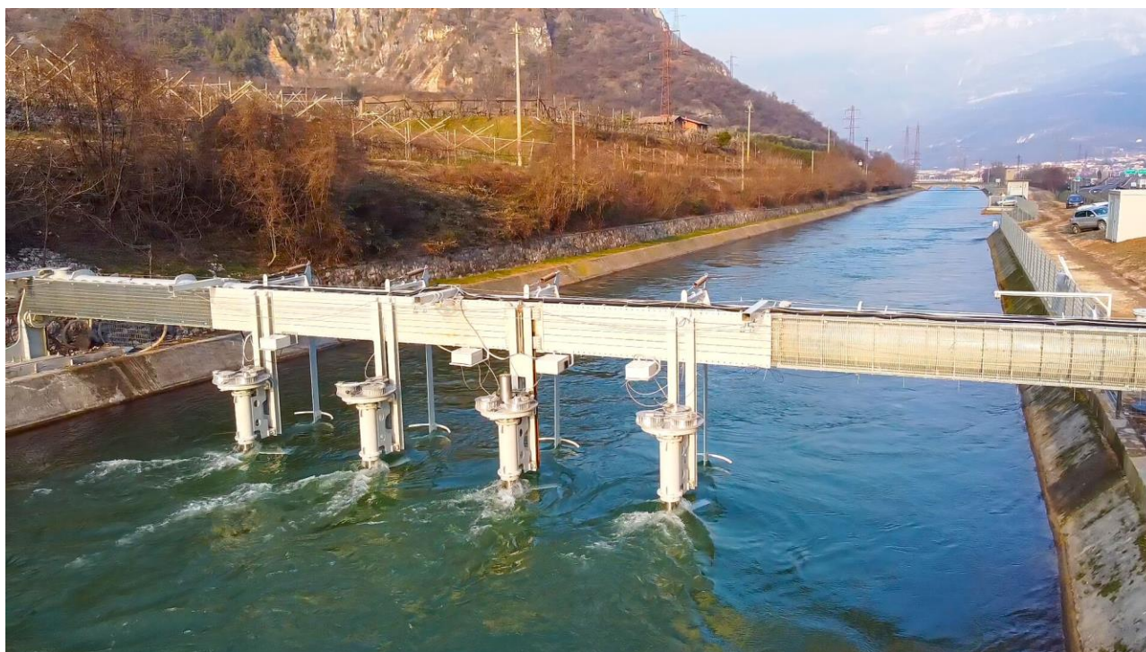
Figure 1. Four aligned VAWT crossflow hydrokinetic turbines installed in a uniform canal configuration (Reprinted/adapted with permission from Ref. [20]. 2023, HE Powergreen S.r.l.).
