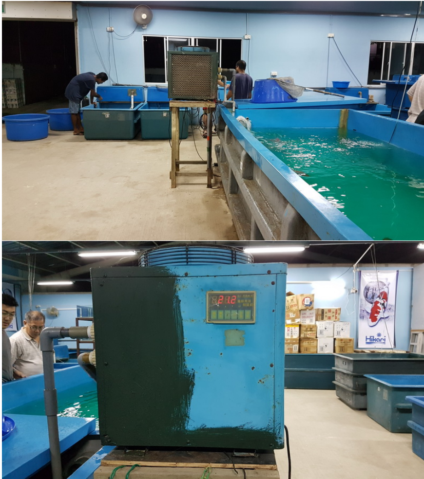
Figure 2.4: An example of a water cooling unit, on Diamond Koi farm. This is used for the koi that had just been imported. (Taken April 28 th 2017)
