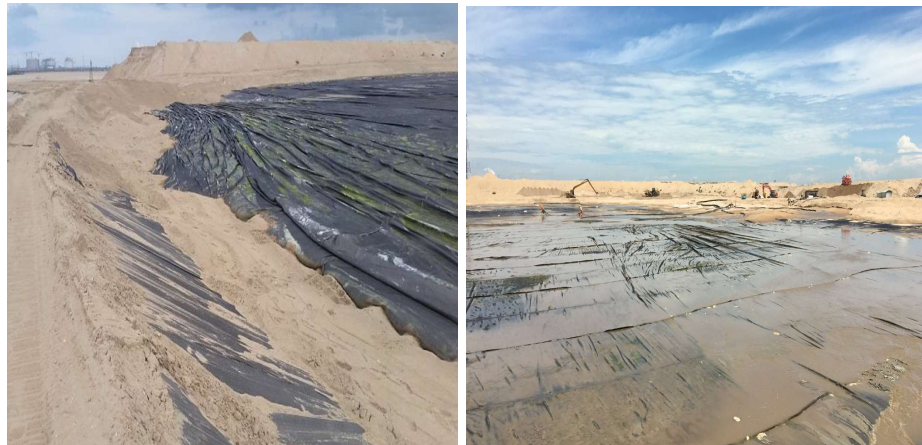
Figure 6.33 Placed geotextiles not in tension
