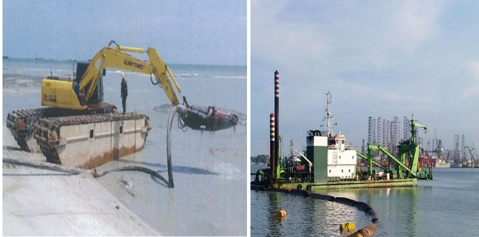
(a) Excavator installed with BELL 200 Pump (b) Cutter suction dredger (CSD)
