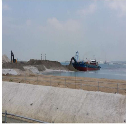
Figure 6.6 Raising containment bund from seabed using conveyer belt barges
