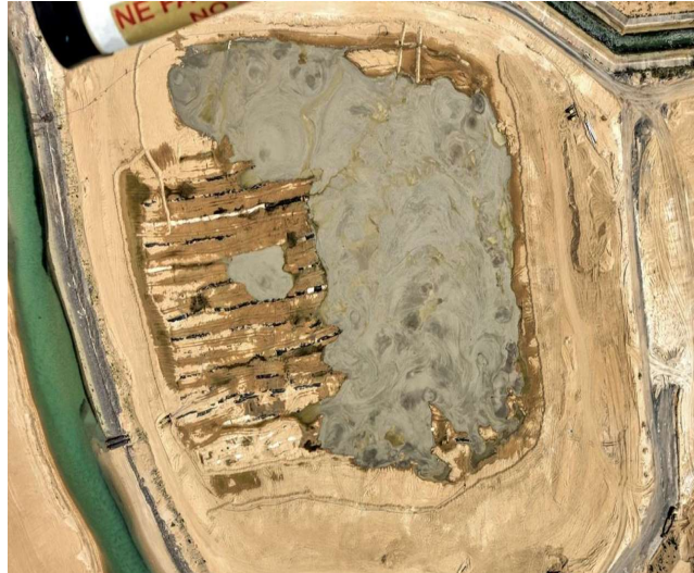
Figure 6.52 Aerial view of the coverage of the slurry from the working platform failure
