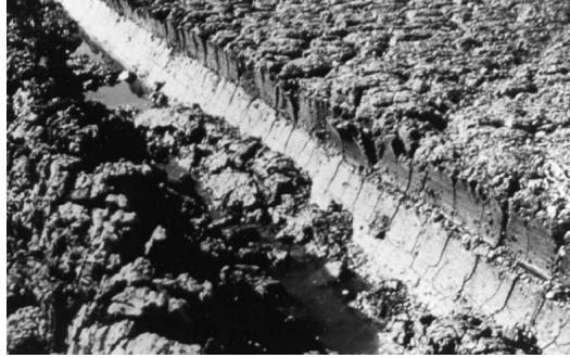
Figure 2.29 Cut trench on clayey sediment surface by rotatory trencher (US, 2015)
