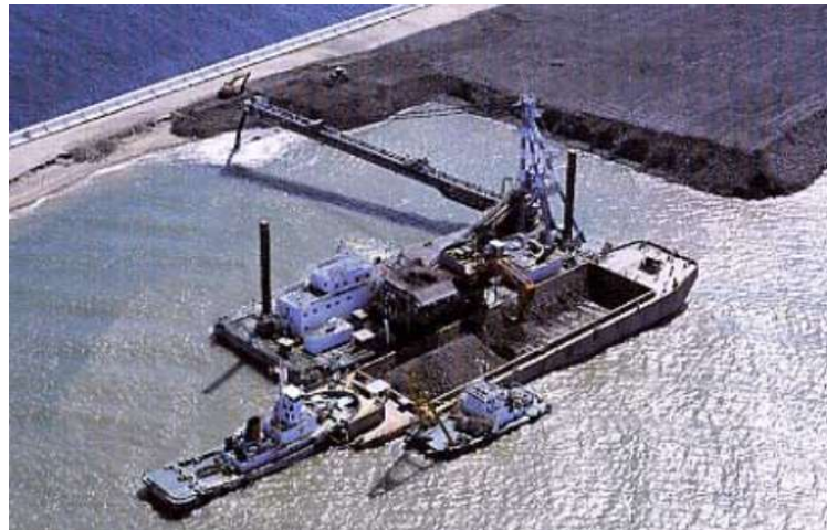
Figure 2.14 Reclaimer barge placing of fill at shallow waters (Kanmon, 2017)
