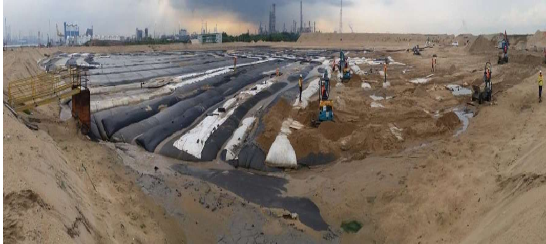
Figure 6.42 Photo showing dry sand placement across geotubes with light equipment
