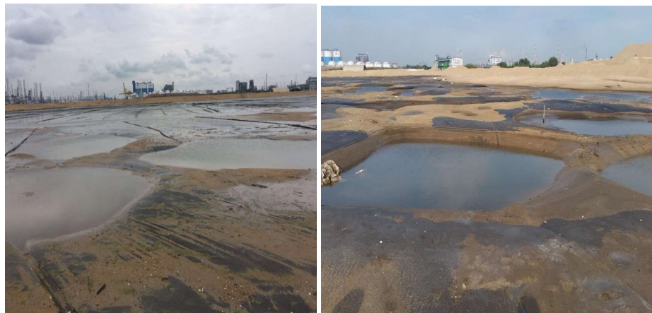
Figure 6.34 Geotextiles pockets containing sand
