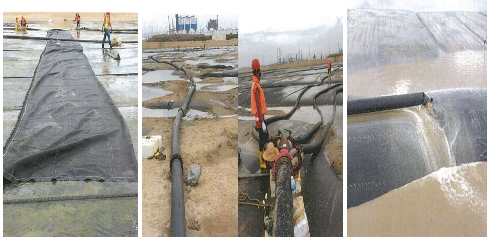
Figure 6.38 Sequence of filling up geotubes using sand
