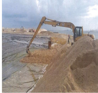
Figure 6.31 Initial sand placement from the sides of containment bund
