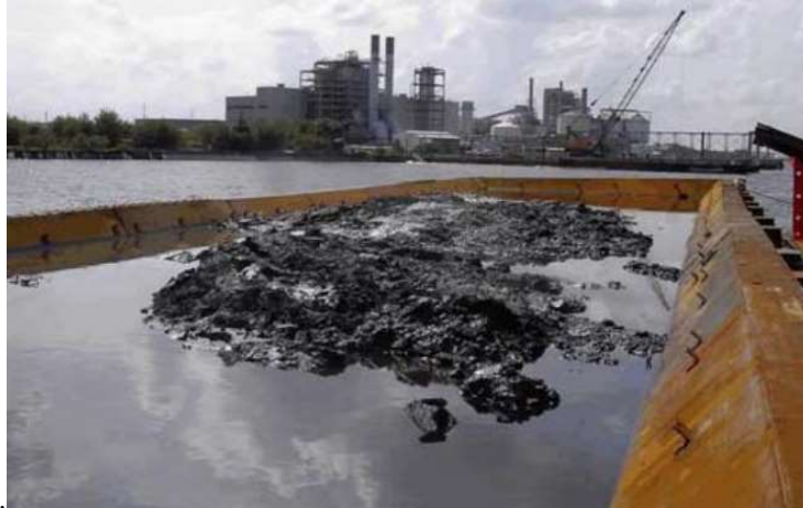
Figure 2.9 Semi-lumpy mechanical dredged seabed sediments (Welp, 2006)
