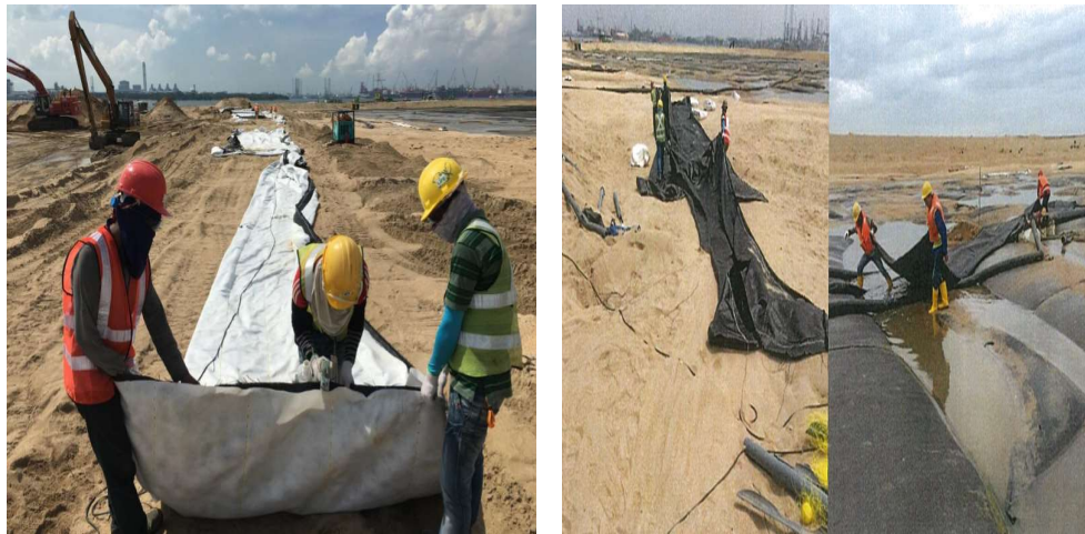
Figure 6.37 Geotube preparation and placement over geotextiles
