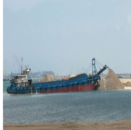
Figure 6.6 Raising containment bund from seabed using conveyer belt barges
