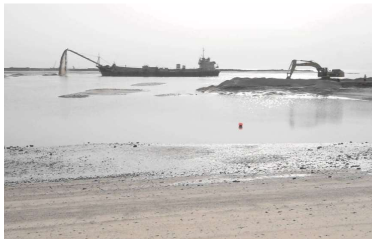
Figure 2.15 Pelican barge discharge fill materials in shallow waters (Kwt, 2015)
