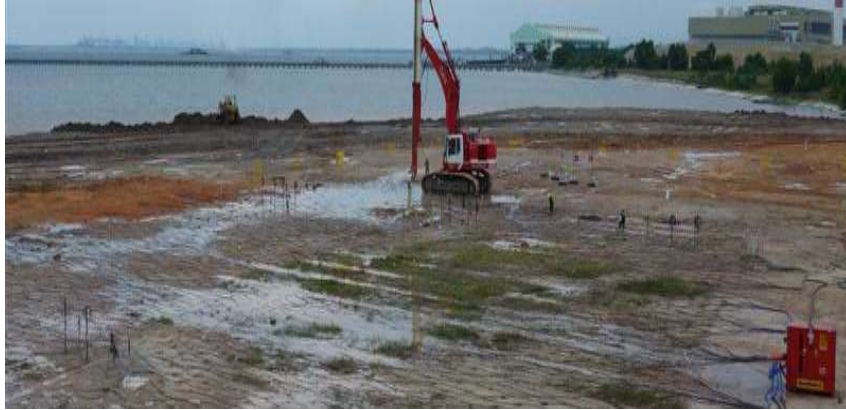
Figure 5.15 Setup of the membraneless vacuum preload system at trial site
