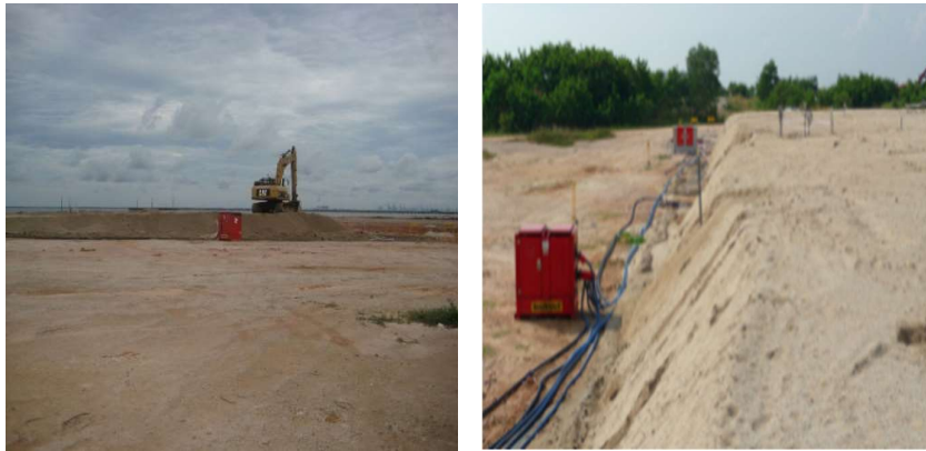
Figure 5.23 Surcharge placement during vacuum operations and final surcharge elevation
