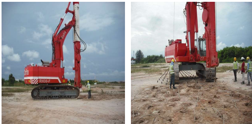
Figure 5.16 Installation of the modified drains in triangular pattern
