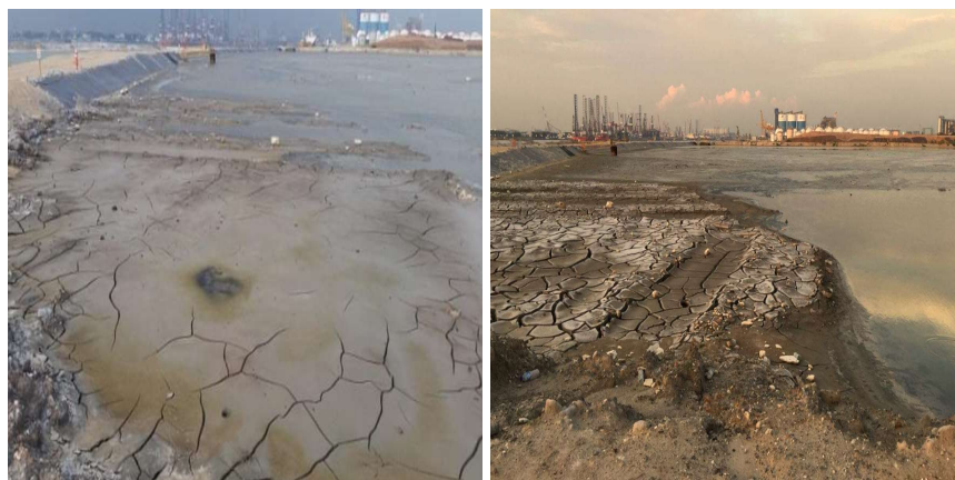
Figure 6.20 Development of the surface desiccation over time at the side of the containment bund and water ponding at the centre surface of the confinement facility
