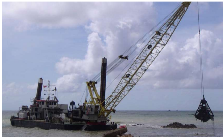
Figure 2.11 Grabbing of seabed materials using grab dredger (Boskalis, 2017)
