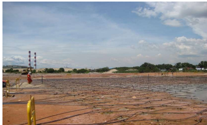
Figure 5.22 Worker checking for vacuum leakages during trial vacuum pumping
