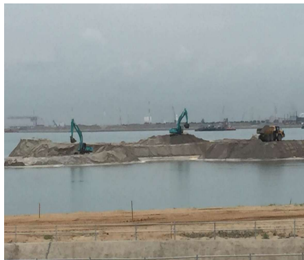
Figure 6.7 Raising and trimming containment bund to final elevation using land based equipment
