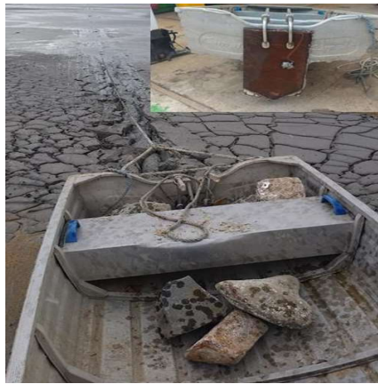
Figure 6.21 Forming shallow trenches across the surface of the desiccated surface layer
