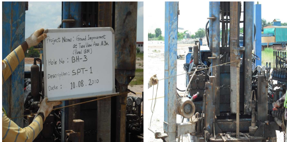
Figure 5.3 Standard penetration test carried out in borehole 3
