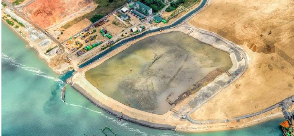
Figure 6.18 Aerial view of the confinement facility after infilling works were completed
