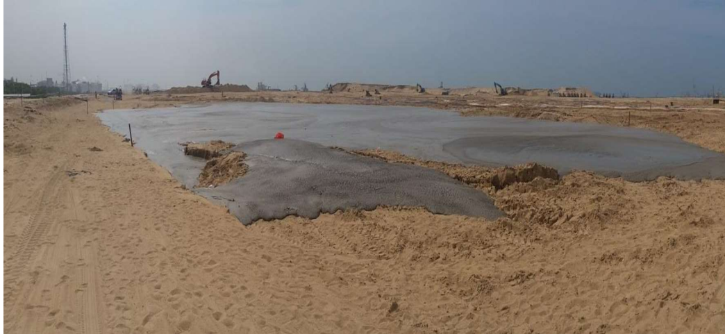
Figure 6.46 Photo showing enlargement of the slurry coverage on day 2
