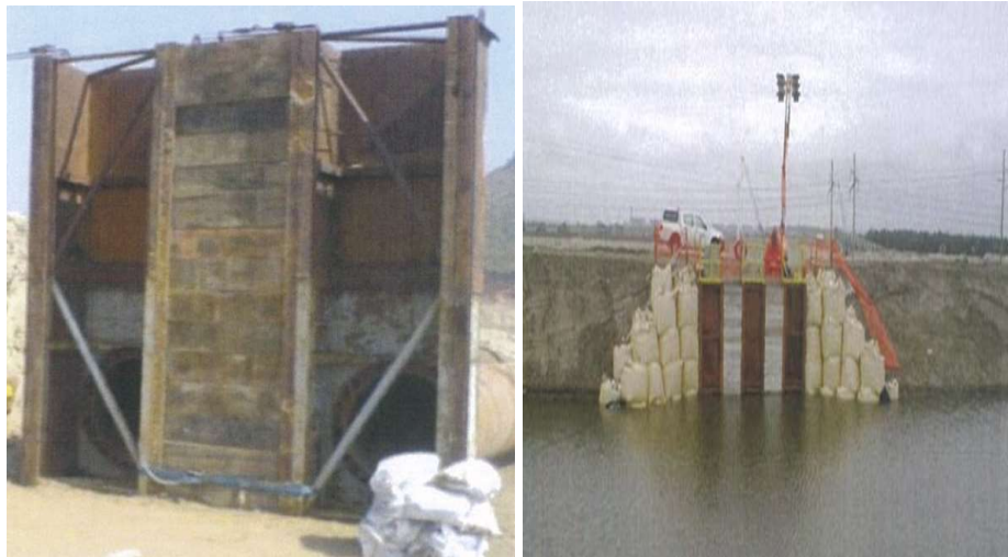
Figure 6.12 Photo showing weir box unit before and after installation
