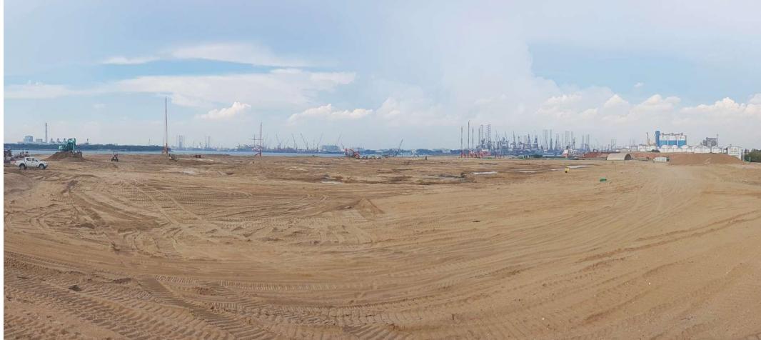
Figure 6.44 Photo showing completed placement for the first layer of sand
