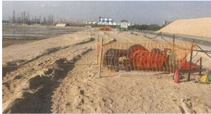
Figure 6.25 Typical installed winch used for the pulling of geotextiles
